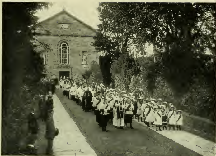
PARISH CHURCH, DONERAILE
